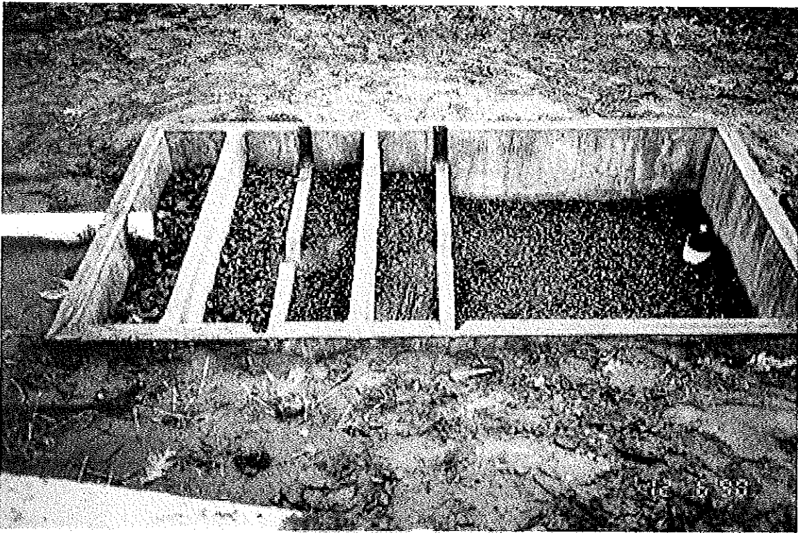
Figure 1: Prototype pretreatment unit under construction.
